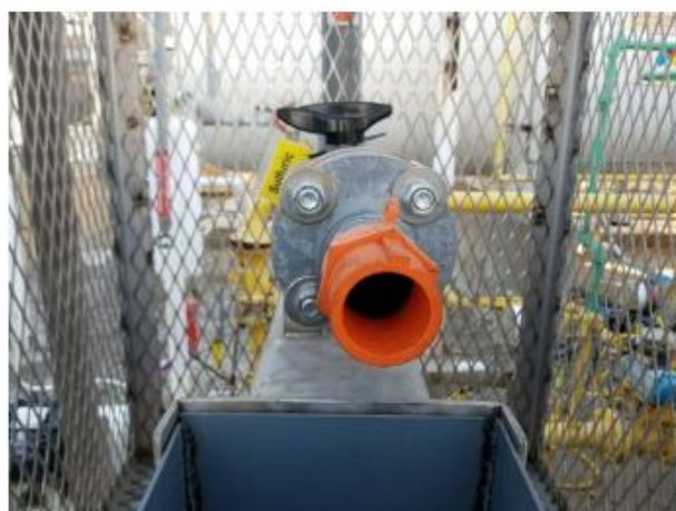
Figure 18. New coupling on the Mod B sulfuric acid fill line (Source: MGPI)
