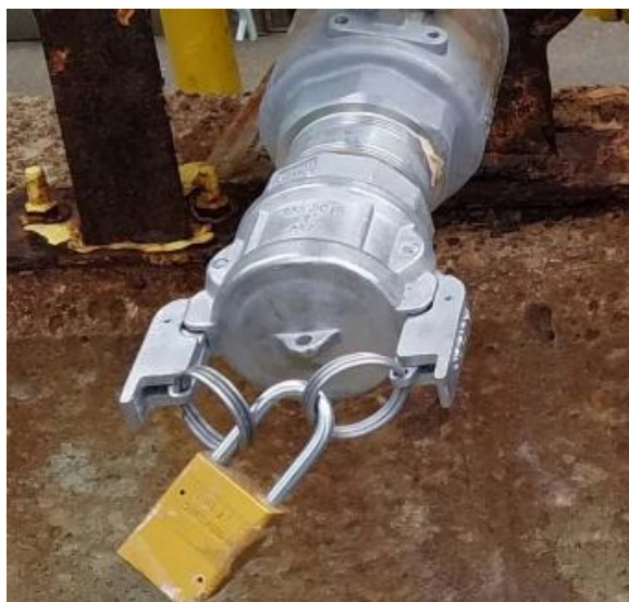
Figure 5. A locked cam lever dust cap on a fill line at Mod B (Source: CSB).
