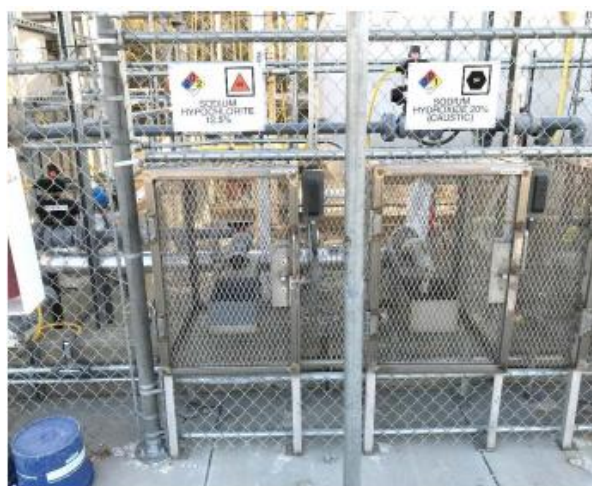
Figure 19. Separation of unloading connections with secure cages around connection points at Mod B (Source: MGPI)
